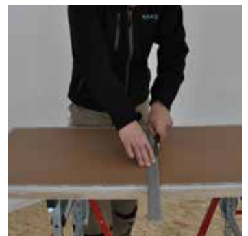
CUTTING THE BOARD TO SIZE
