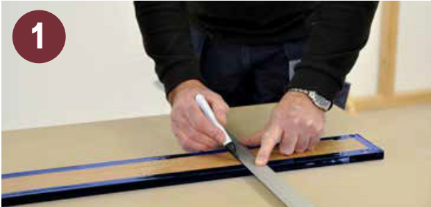
1 MEASURING AND MARKING THE CUTTING LINE
