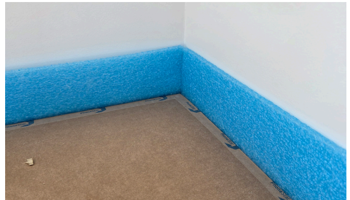
Butt-joint the Woodland insulation strip in the corners
