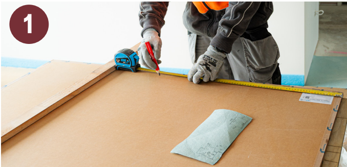
1 MEASURING AND MARKING THE CUTTING LINE
