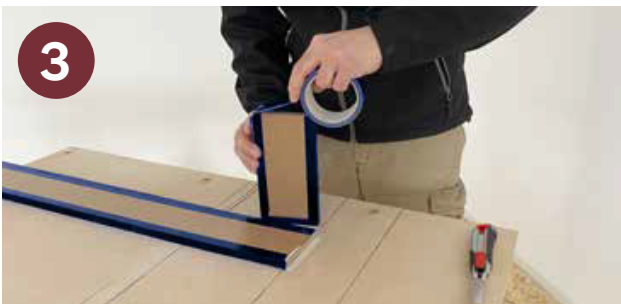
3 MASK THE DECOUPLING STRIPS
