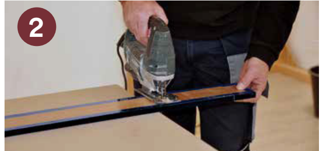
2 CUT THE DECOUPLING STRIP TO SIZE
