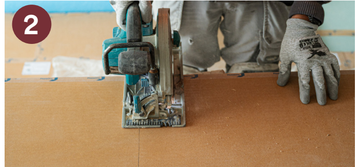
2 CUTTING THE BOARD TO SIZE
